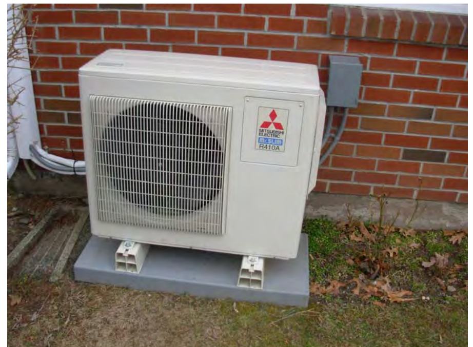
16. Heat pump HVAC system exterior condenser units
