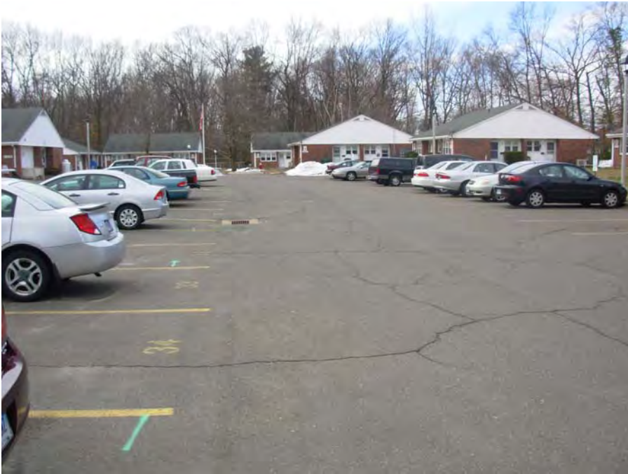
1. Parking area surface cracking
