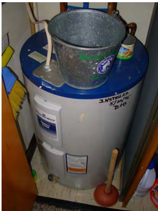
15. Electric DHW tanks serving apartments
