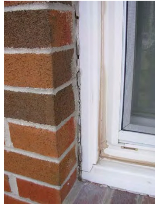
6. Caulking deterioration around window frames
