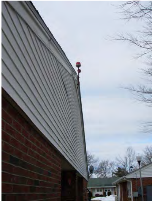
5. Spot vinyl siding bulging, seam separation
