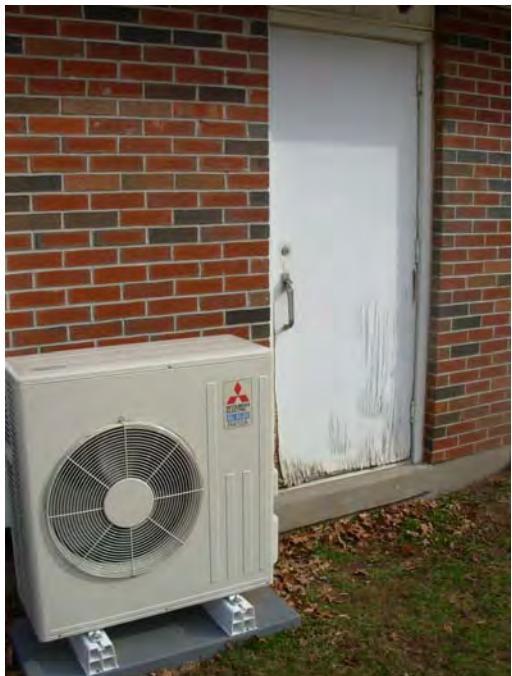
7. Service door deterioration, note Cmnty. heat pump condenser unit
